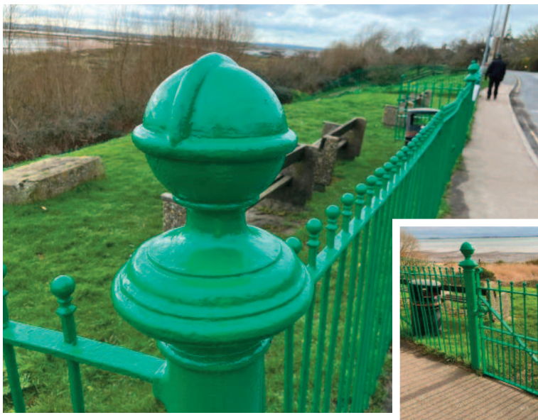
Refurbished fencing at Coastguard's Compound.
