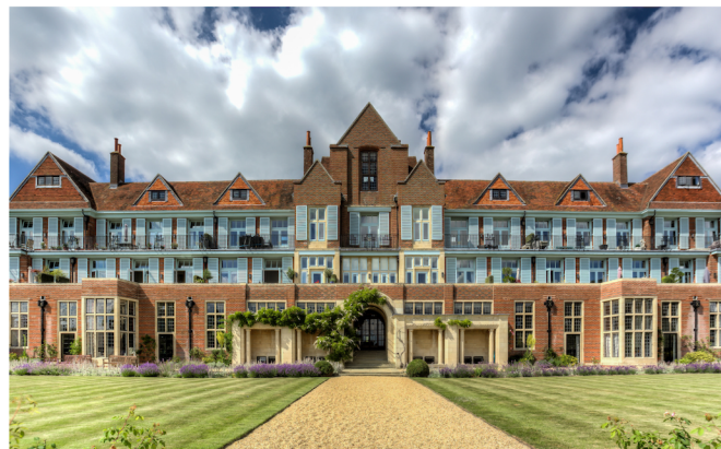
King Edward VII Estate - Mix of Conversion and New Build Housing
