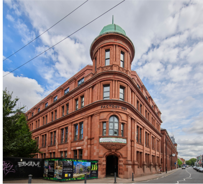
Factory No 1, Bristol - High Street Ground Floor Retail/Commercial Units
